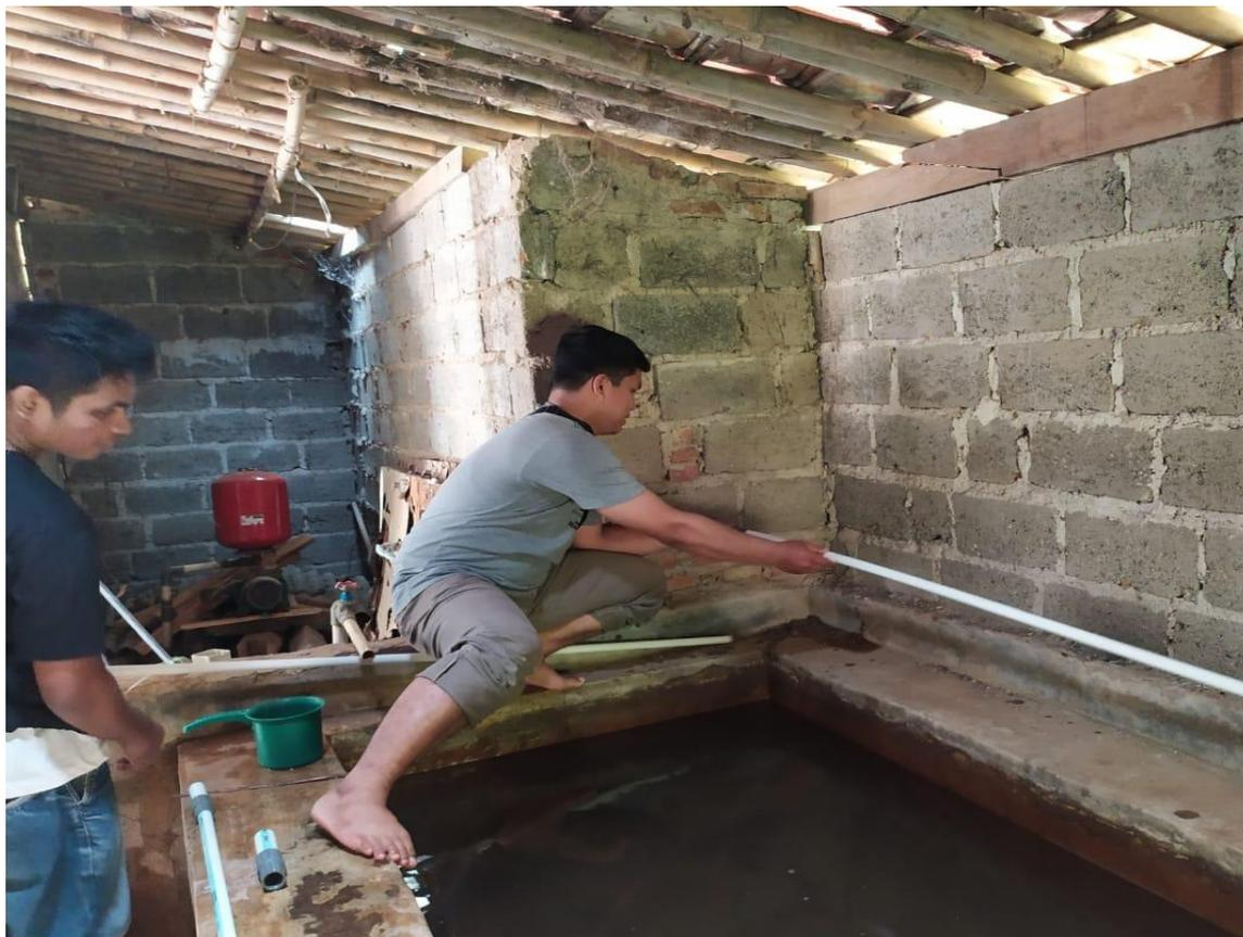
Gambar 11. Proses Instalasi pipa air wudlu
