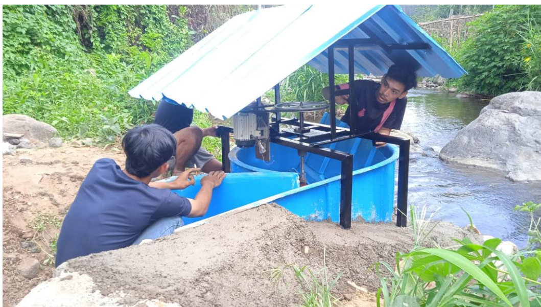
Gambar 6. Hydro Vortex System Chamber (Off Grid Test)
